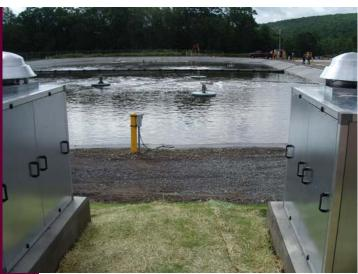
Supported with two small blowers, MAMA added ten new O<sup>2</sup>ctopus<sup>®</sup>. Stainless diffusion units, along with four new Bio<sup>2</sup>Bloc modular fixed film reactors to improve treatment and reduce electrical operating costs. The project was installed in a 3-day period in July 2006, with no down-time to plant operations.
