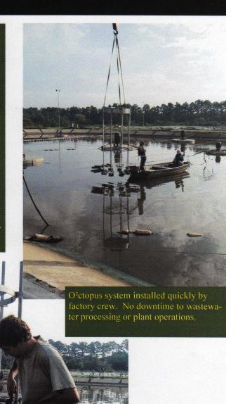
Octopus units installed with 16 diffusers per unit, providing superior oxygen transfer & mixing in a small system footprint.
