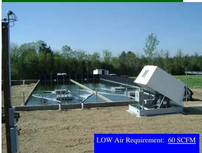
Patented “Dual Diffusion” technology: shore-mounted controls for easy back-flushing whenever necessary.
