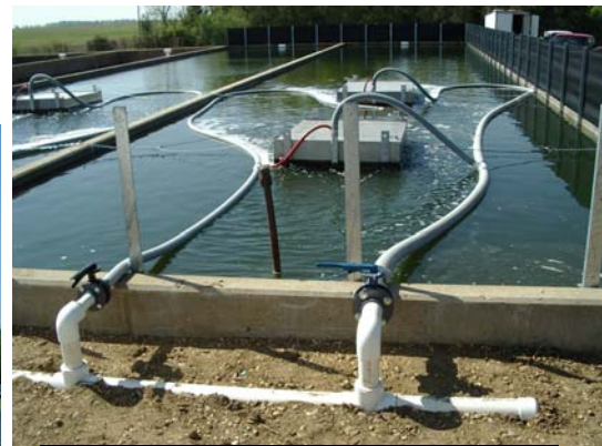
Patented “Dual Diffusion” technology: shore-mounted controls for easy back-flushing whenever necessary.
